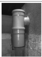
It must be ensured that there is an emergency overflow (> 40 cm²) between pretreatment or buffer tank and SBR tank!
