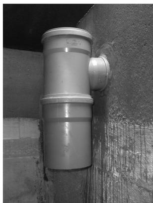
Install T-piece for the overflow between (last) pretreatment chamber and buffer tank as well as for the runout. The level should lie at one height.
