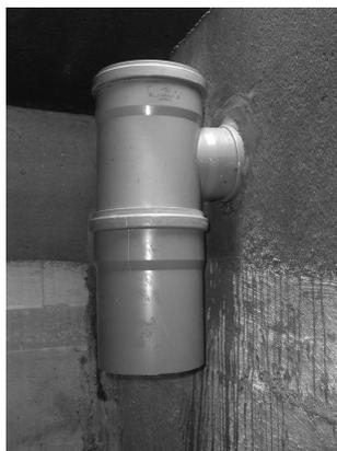
It must be ensured that there is an emergency overflow (> 40 cm<sup>2</sup>) between buffer tank and SBR tank!
